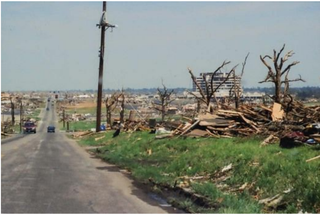
FIG. 10-1 St. John's Regional Medical Center in Joplin, Missouri, after a powerful tornado struck in May 2011.
